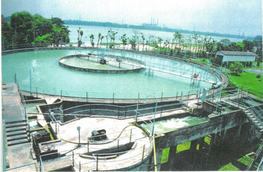
Exhibit 12.1 Serampore Water Treatment Plant showing Parshall Flume, flash mixer and clariflocculator
